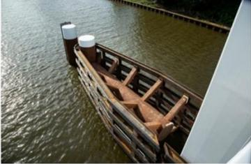
protects the lock or bridge against collision damage
